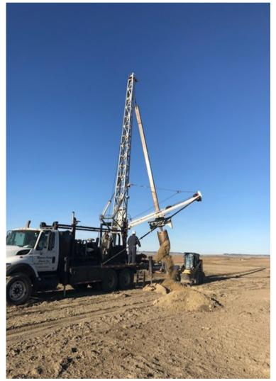
Setting conductor pipe at Govt Kaehne #29-9 well
